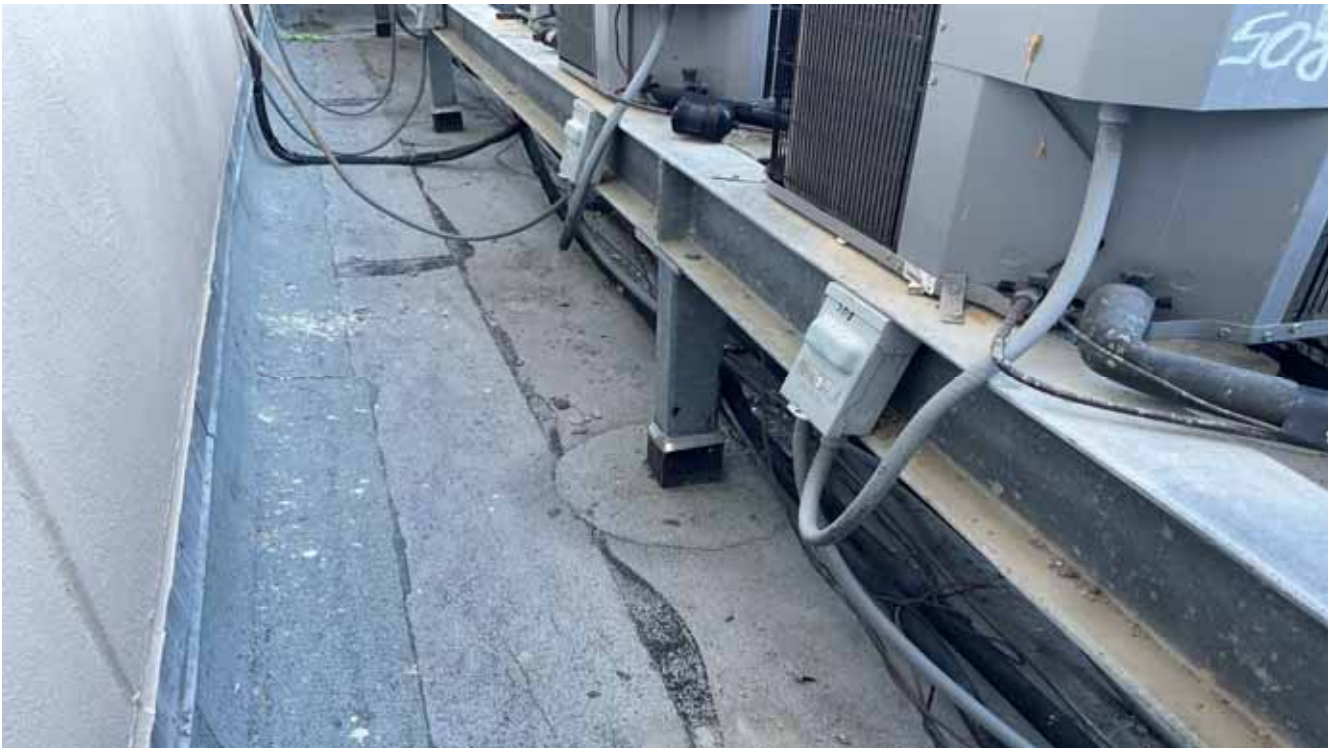
Condo Bldg Roof-2nd Floor
