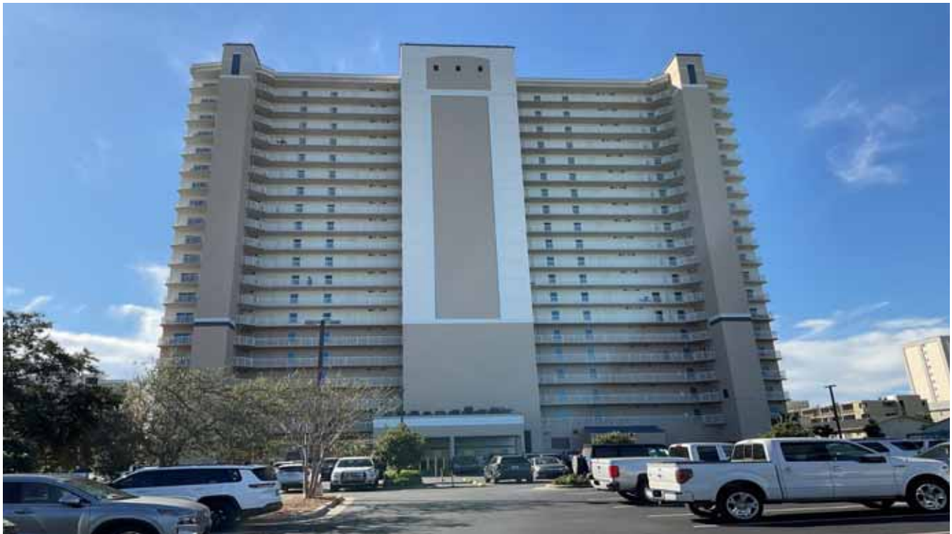
Condo Bldg Elevation, North
