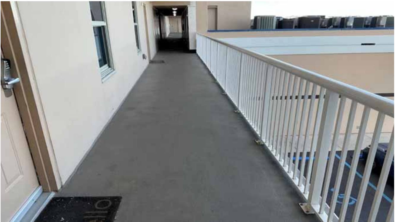
Condo Bldg Typical Walkway
