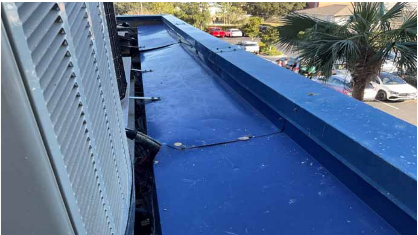
Condo Bldg Roof A/C Conduit Cover-2nd Floor
