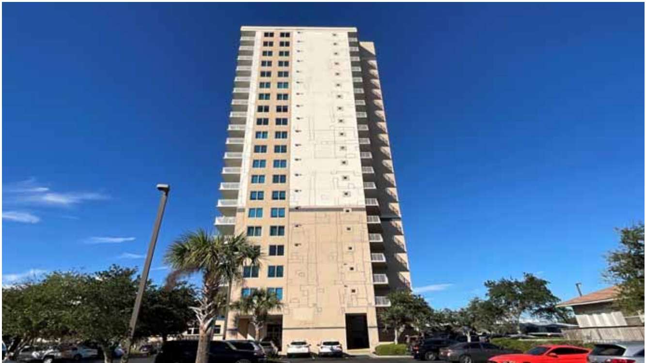
Condo Bldg Elevation, East
