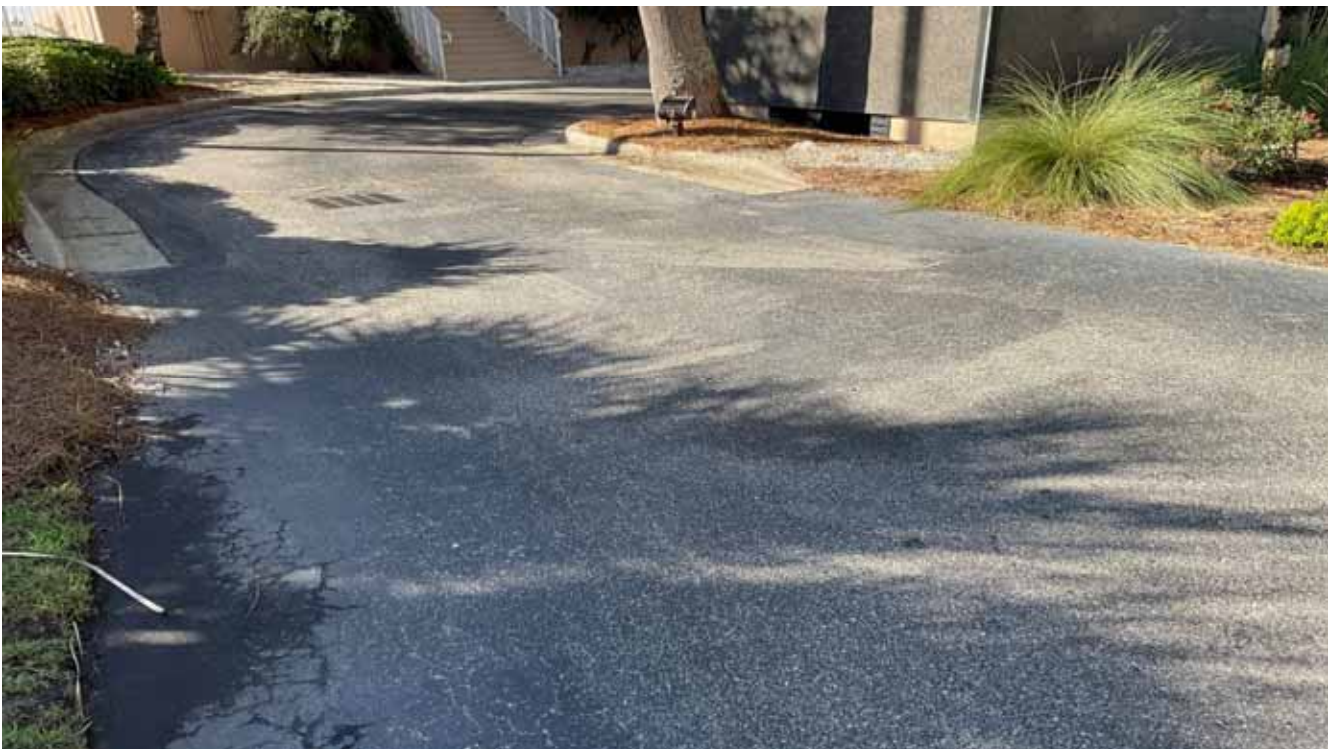
Paving, Asphalt - South Pool House
