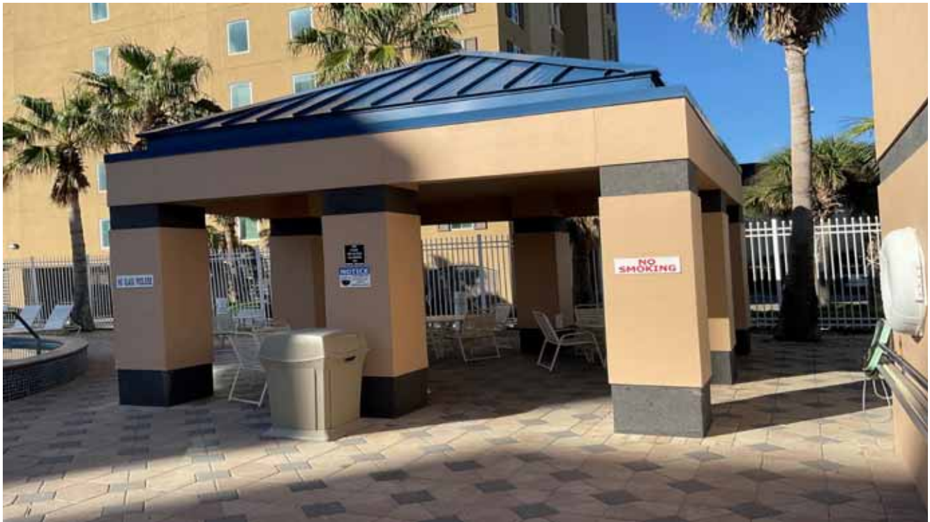
South Pool Area Shelter
