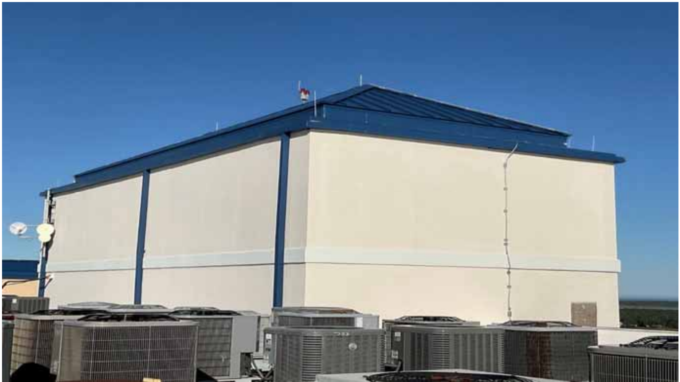
Condo Bldg Roof, Metal
