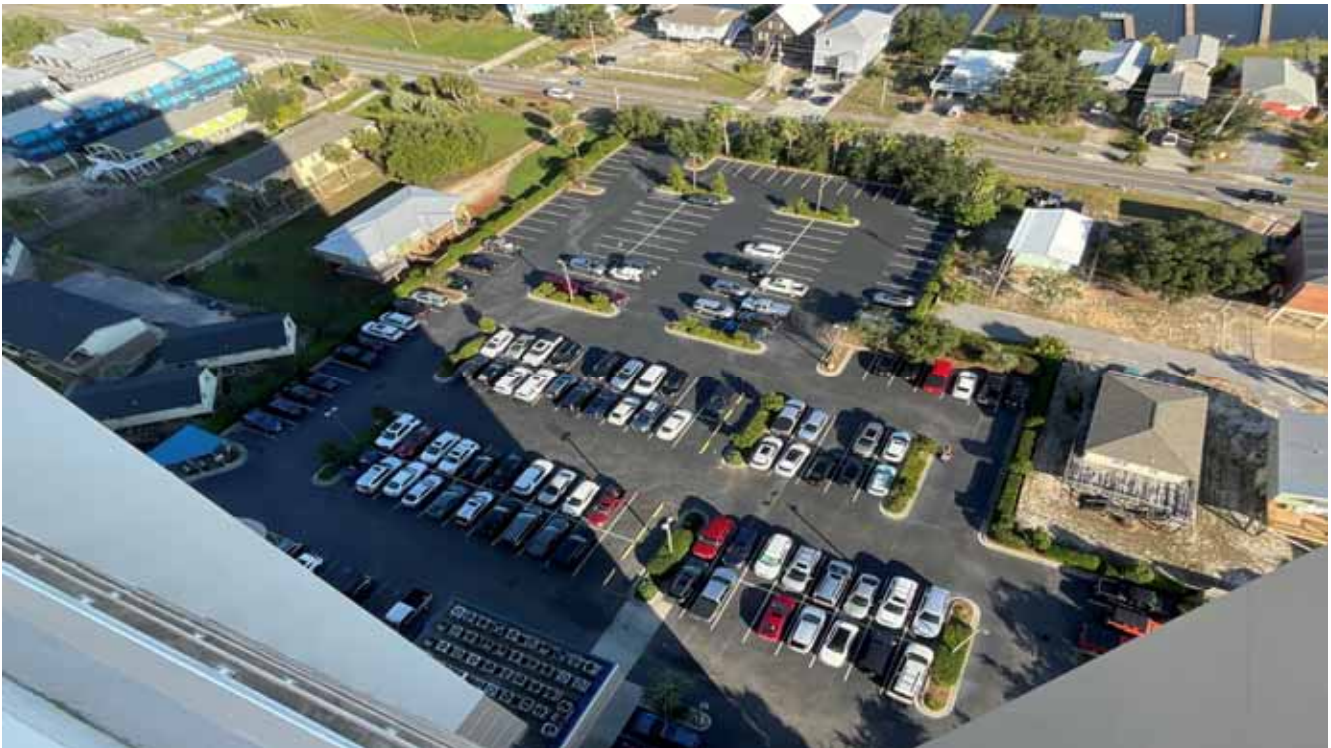
Paving, Asphalt - North Parking Lot
