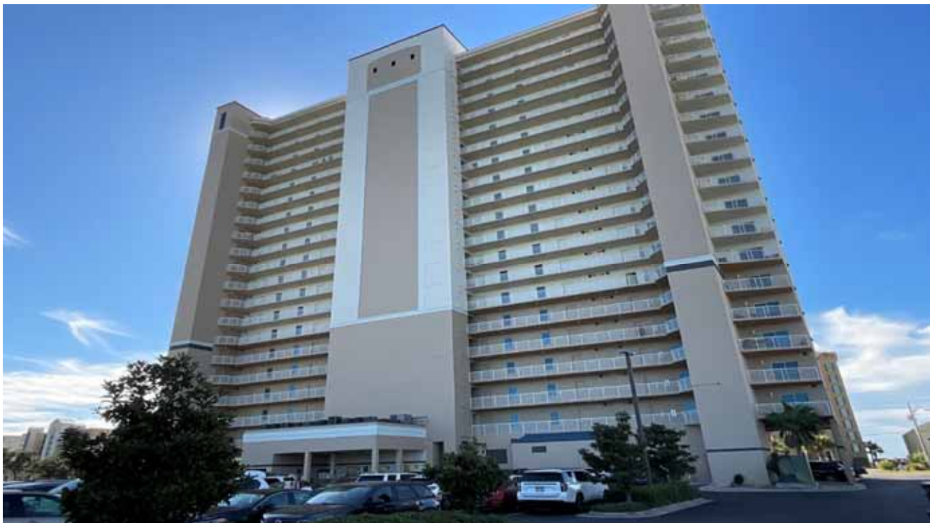
Condo Bldg Elevation, North
