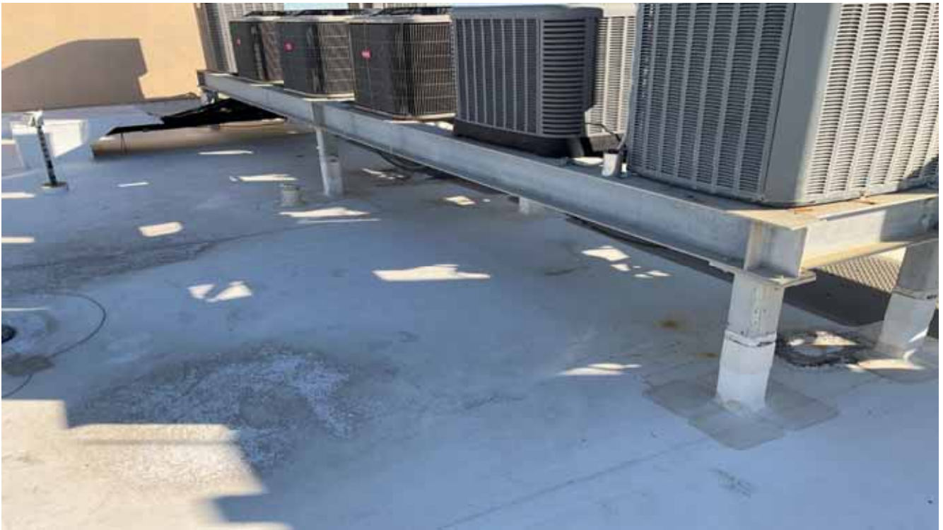
Condo Bldg Roof & A/C Stands
