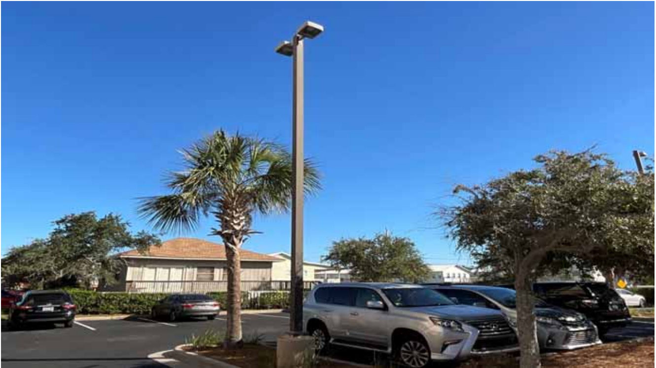
Light Pole - Parking Lot
