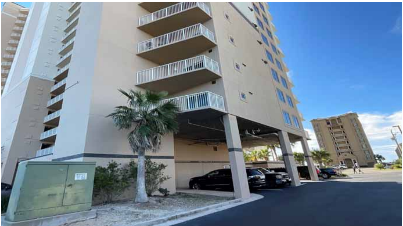
Condo Bldg Elevation, West
