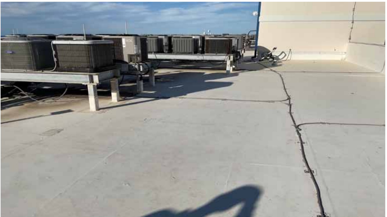
Condo Bldg Roof & A/C Stands
