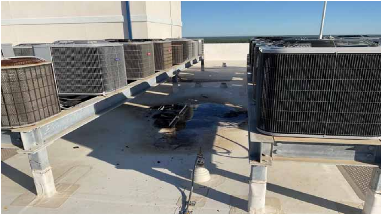
Condo Bldg Roof & A/C Stands
