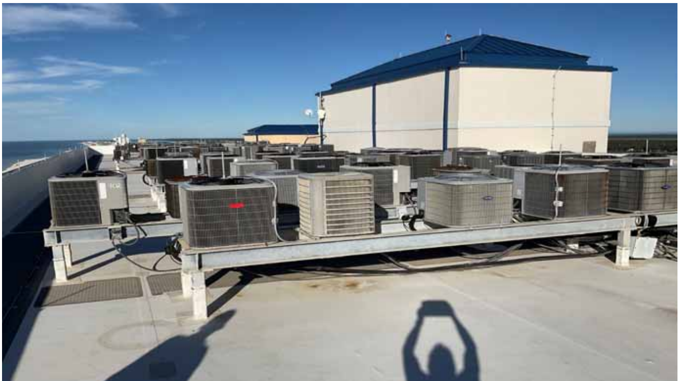
Condo Bldg Roof & A/C Stands
