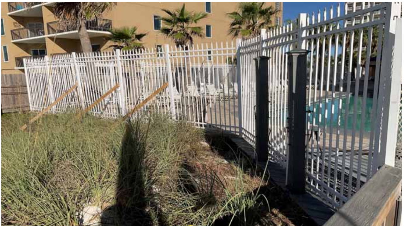
South Pool Area Fence
