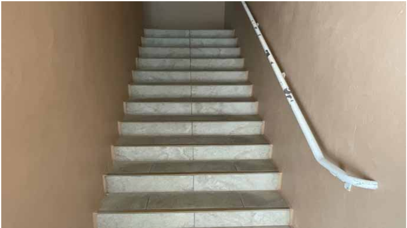
South Pool House Stairwell
