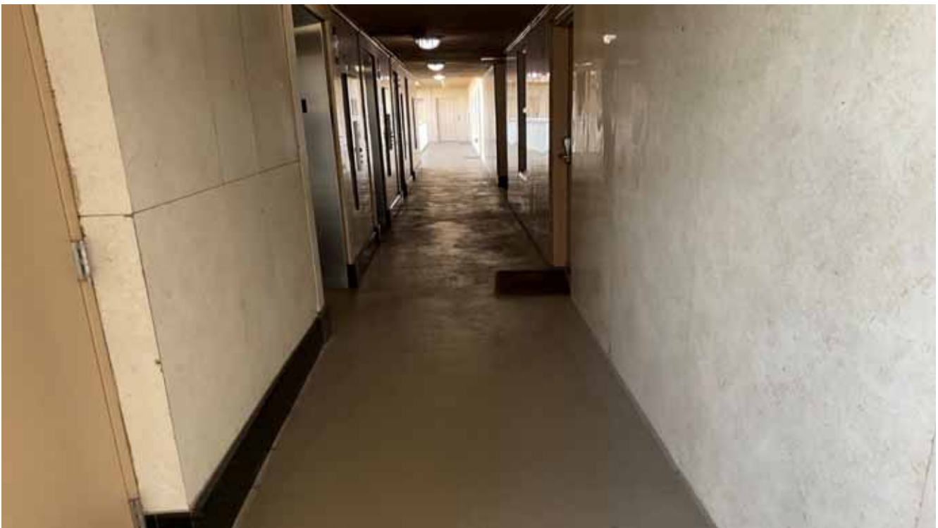
Condo Bldg Typical Walkway
