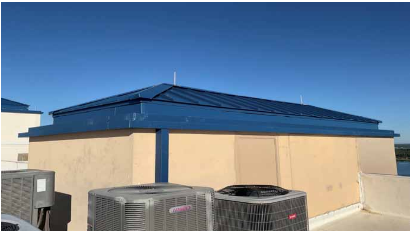
Condo Bldg Roof, Metal
