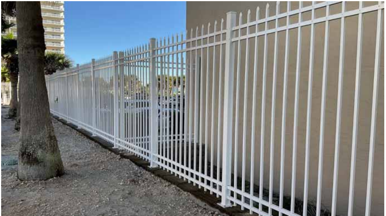
South Pool Area Fence
