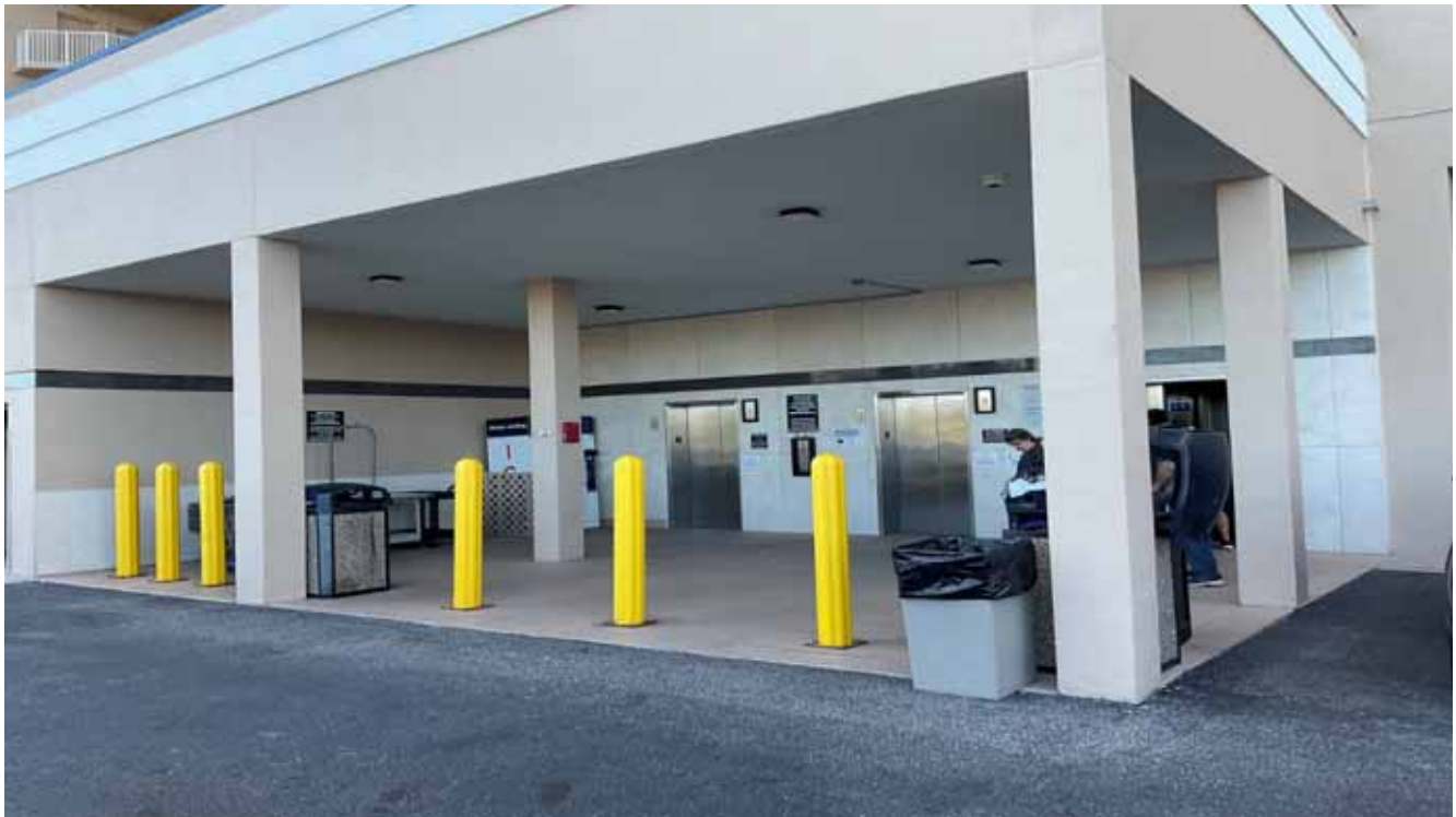
Condo Bldg P Level Elevators
