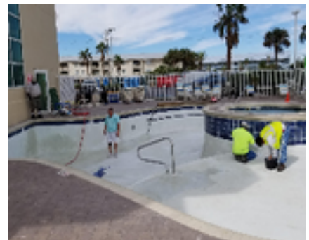
Stain Removal & Grouting
