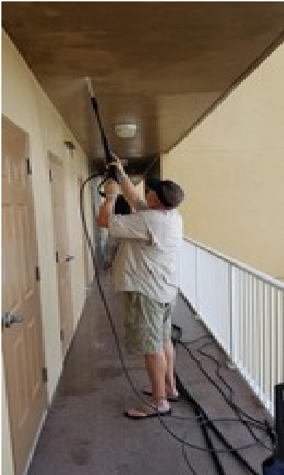
Aaron Powers pressure washing a breezeway ceiling.
