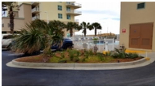
We plan to dig a "dry well" or French Drain here, remove the Saw Palmettos, and use a river rock ground cover here, too!
